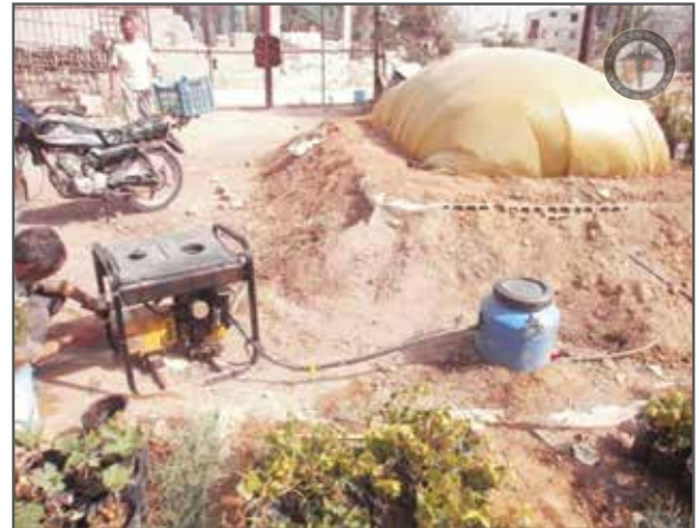
Biogas pit, part of a SAMS/SAEA sustainable energy project, in operation in besieged Douma in Eastern Ghouta.
