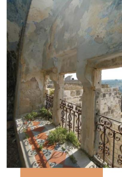
According to Nurjihan Riyad, a preservation architect working with UNDP, the stone used for restoration work should be softer than the stone of the original building. Adding harder stone to a building will put stress on the original, softer stones and cause them to deteriorate more rapidly. In the West Bank, stone from Jema'een is particularly good, she says, because it is soft and weathers to a light golden color, "achieving a harmony within the restored facade."
