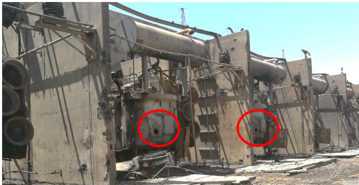
At Western Mosul's main power station, heavy calibre rounds were deliberately fired into a block of power transformers filling the basement of the building below with up to 3 metres of potentially toxic transformer oil © UNDP
