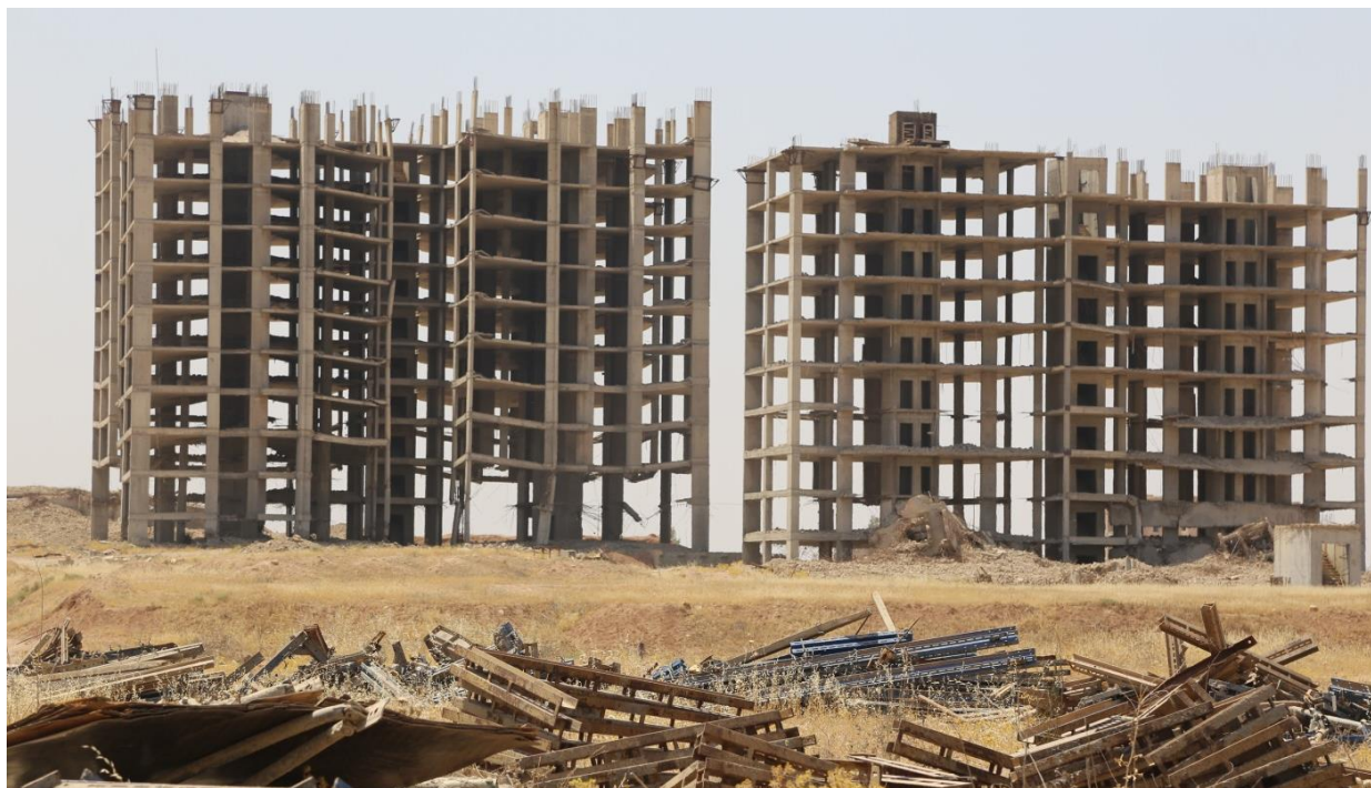
The foundational pillars of these buildings were blown-up by ISIL, necessitating their demolition © UN Environment
