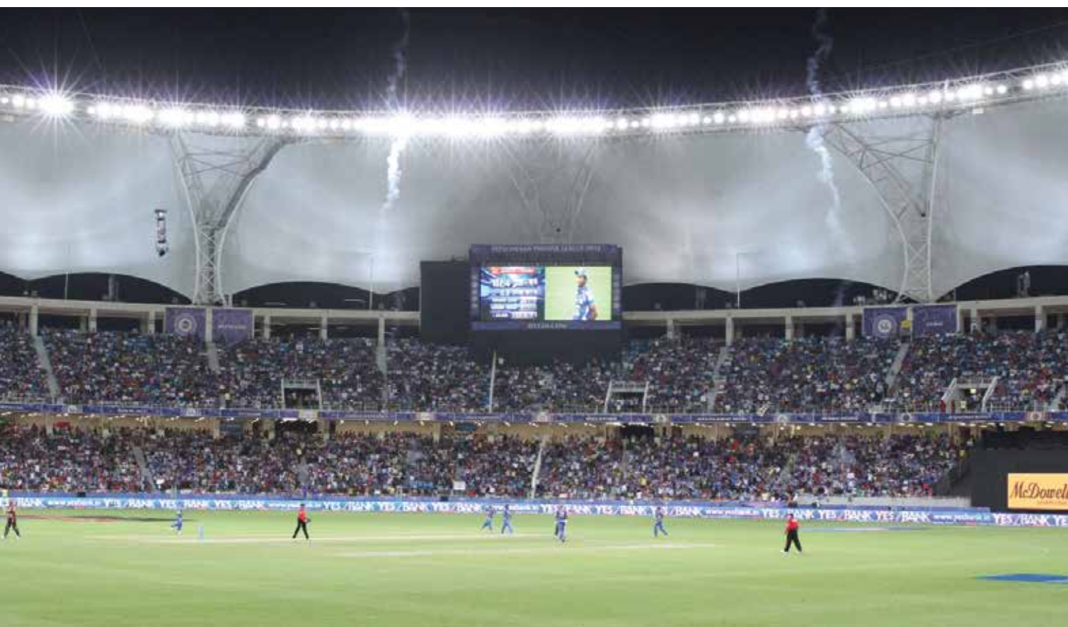
Dubai International Stadium at Dubai Sports City
