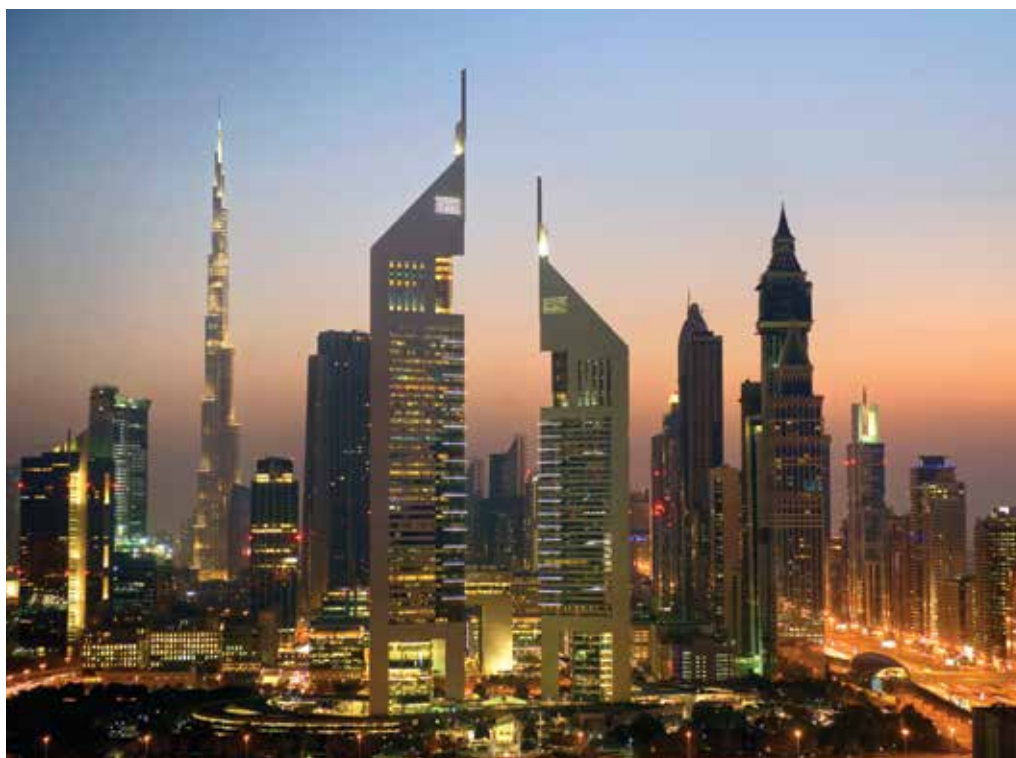
Jumeirah Emirates Towers
